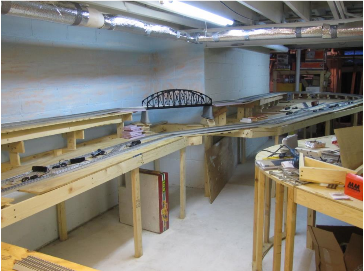
Facing West –Southwest: Center Canyon; (Low line to be double arch bridge (two arches per mainline))
