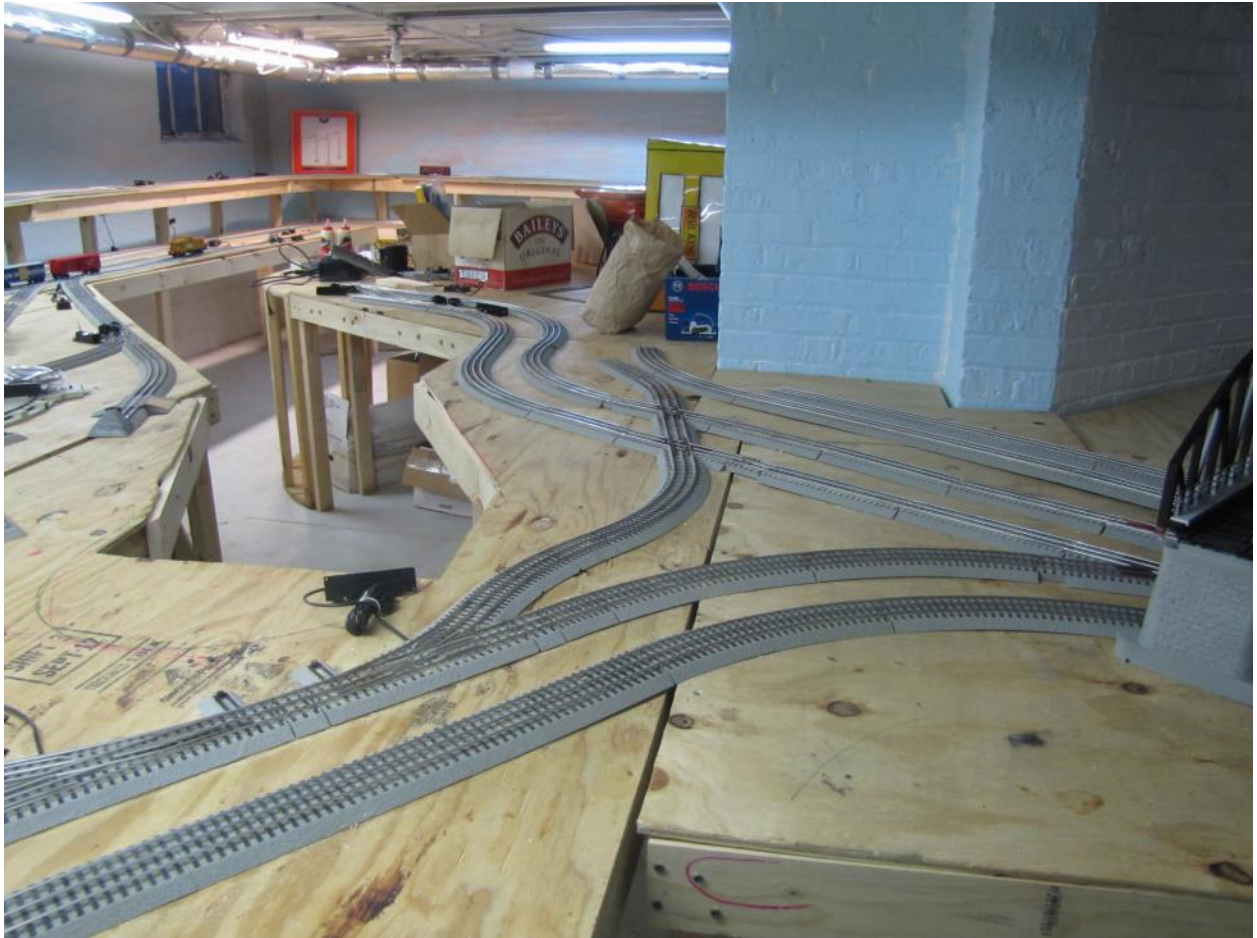
Facing South: Access Aisle (20-inch minimum); East City Approach; City Industrial Lead with 2 x 45° Crossovers. (Note: City to be located where material boxes are located)
