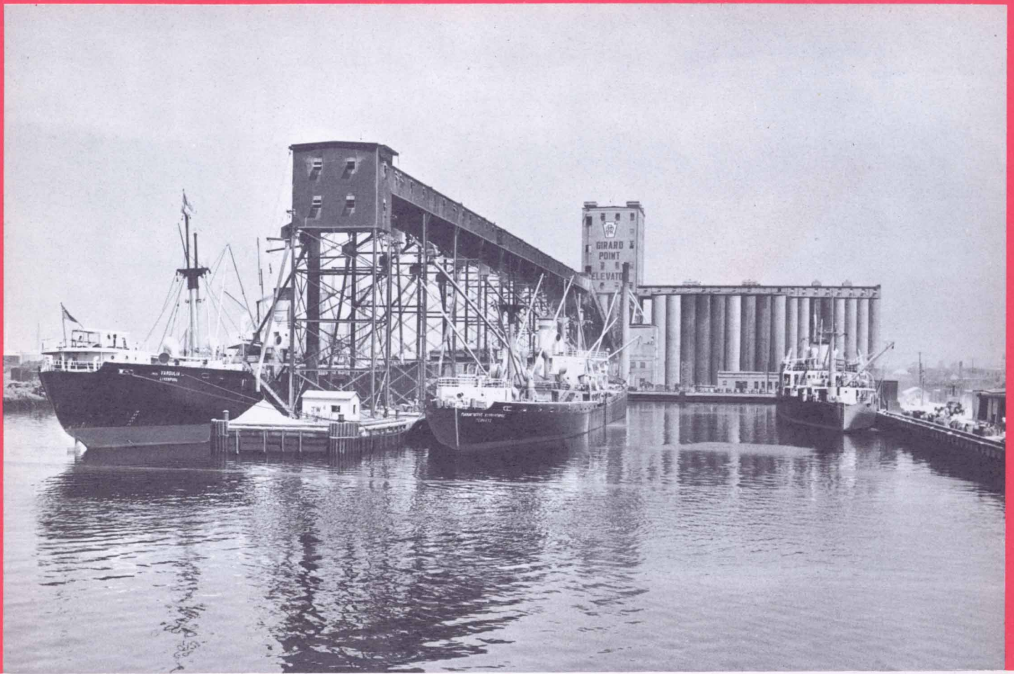
PENNSYLVANIA RAILROAD GIRARD POINT ELEVATOR , capacity 2,225,000 bushels. The elevator is equipped with all modern facilities for handling grain. Three vessels can be berthed simultaneously at this facility.
