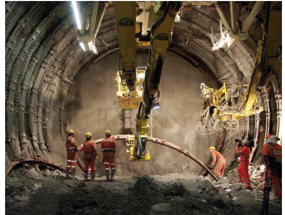
Work on the new Gotthard tunnel has considerably progressed
