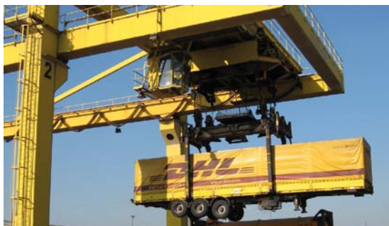
Gantry cranes are the main transfer equipment in bigger terminals
