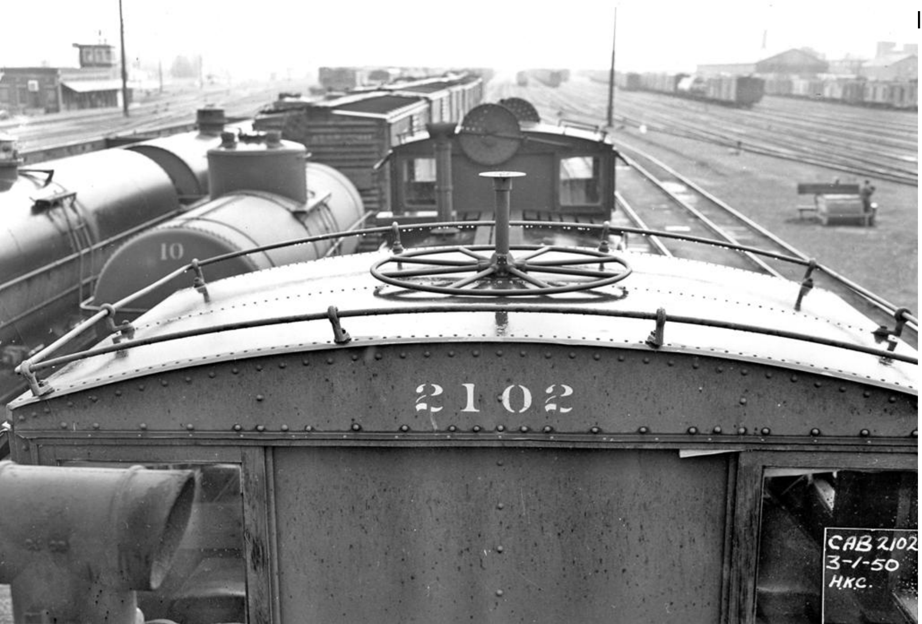
Cupola mounted "wagon wheel" radio antenna
