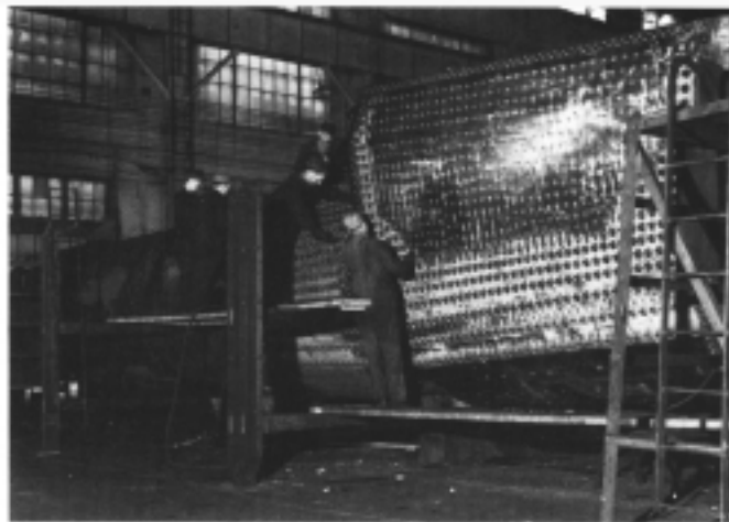
Made July 18, 1941, showing fabrication of firebox and boiler shell. The assembly is turned upside down in the photograph to enable easy access to the outside of the firebox by the boilermakers, who are shown in the picture applying flexible staybolt caps around the throat sheet, utilized as a connection between the firebox and second boiler barrel. Photo from N-S files. Caption by A. M. Bixby, Sr.
