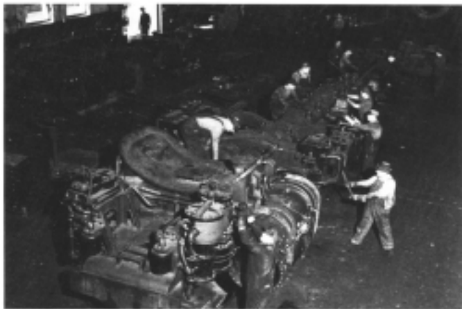
Made July 14, 1941 at N&W East End Shops in Roanoke, Va., showing cast steel steam locomotive "Bed". This huge one piece casting includes the entire locomotive frame, the two cylinders, various brackets for mounting of auxiliaries and a large support for mounting of cab. Note the 8½" cross compound air compressor mounted at left front of pilot beam, with workman connecting piping to carry air throughout the locomotive and train behind. The cylinder saddle appears just behind the air compressor, where the front end of the boiler or smokebox will seat. The cast steel "locomotive bed" was a great improvement in steam locomotive construction. Another bed frame appears at top left of photograph, showing cylinders prior to application of heads. Photo from N-S files. Caption by A. M. Bixby Sr.
